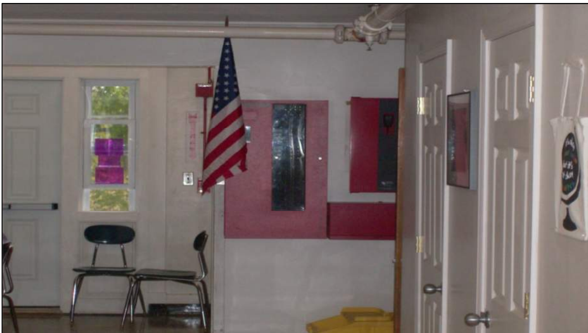
Fire alarm panel in original section of school.
