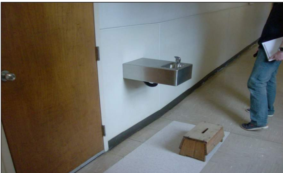
Drinking fountain extends out into corridor and creates an obstruction.
