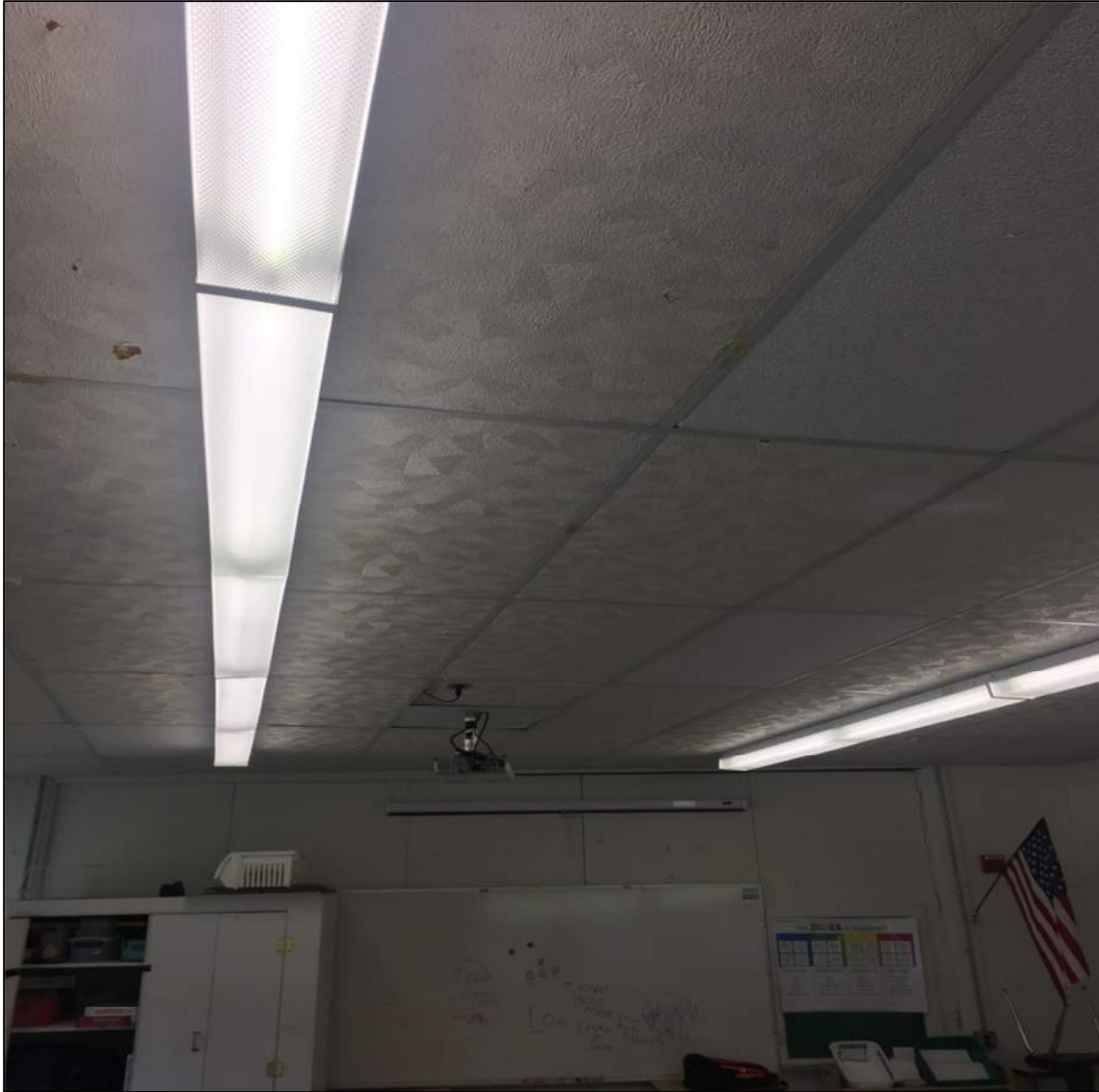
Drop ceilings need to be replaced and upgraded.
