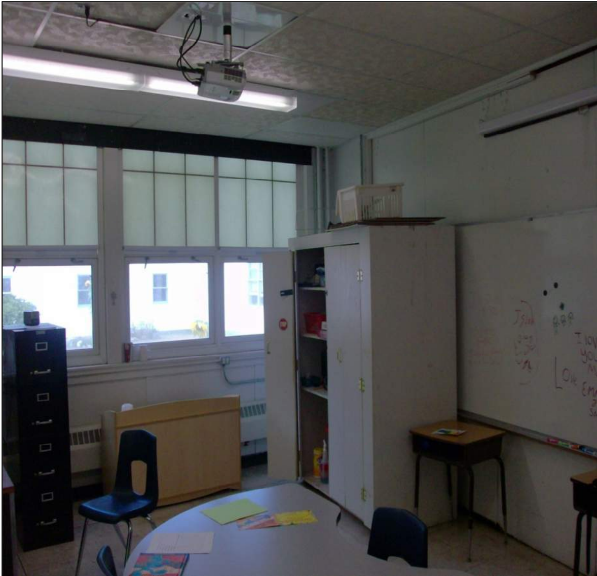
Old hopper-style windows with Kalwall panels above.
