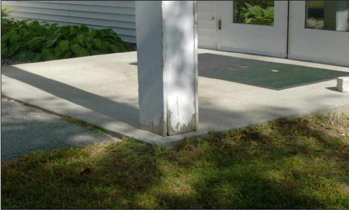
Posts at west entrance needed paint and showed signs of wood rot.
