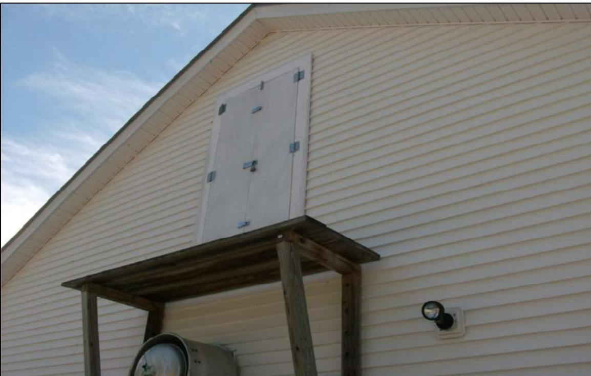
Platform to access HVAC unit over kitchen. No handrail makes this particularly dangerous.
