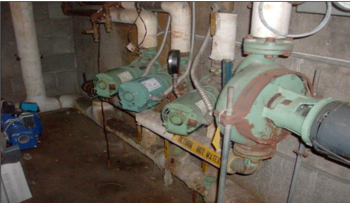
Two of three circulating pumps should be upgraded.
