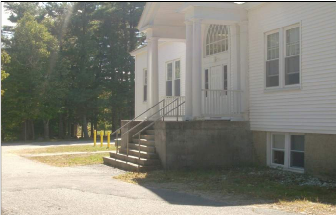
Former main entry on east side. Stairs are non-compliant.
