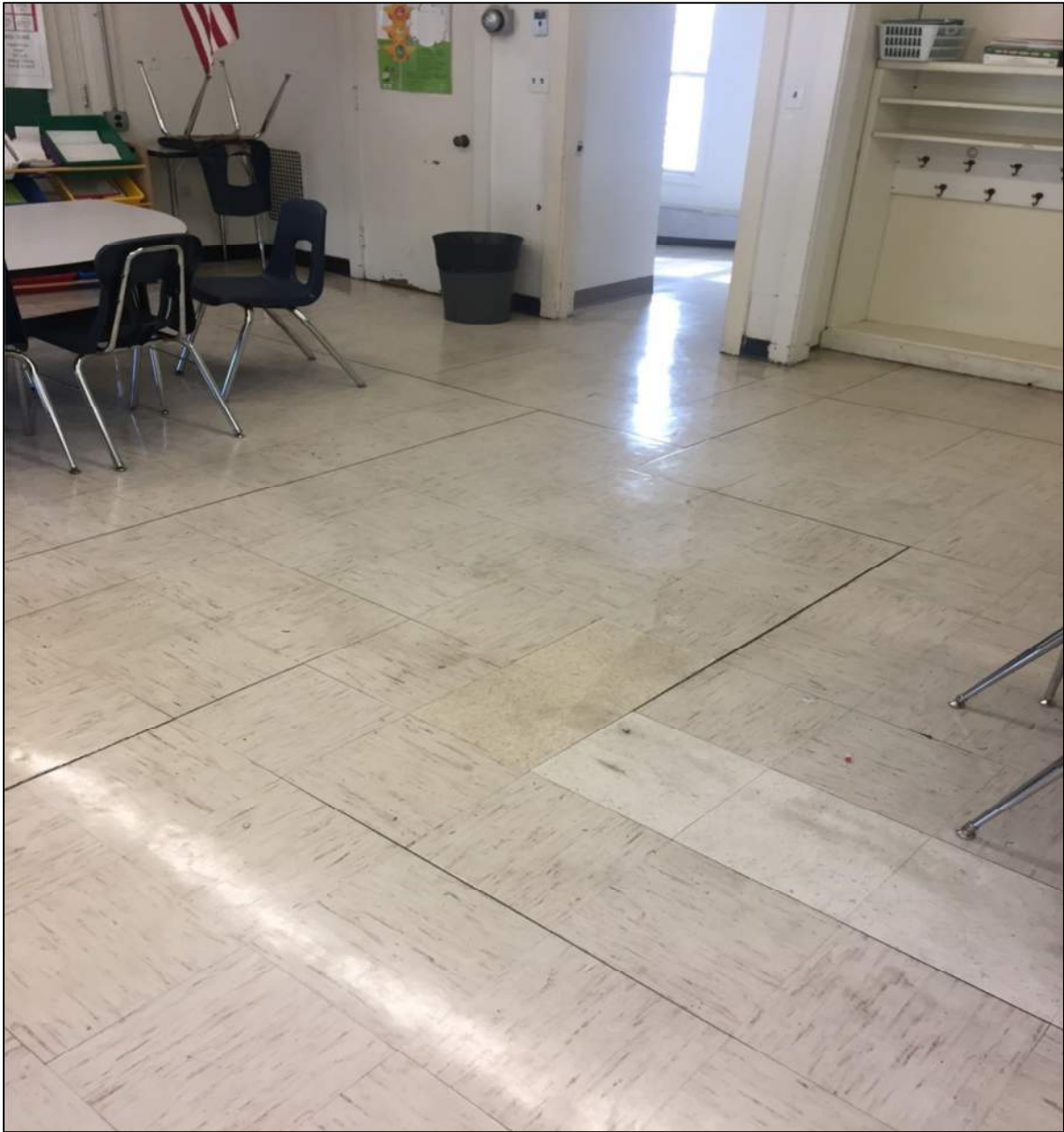
VCT flooring in 1950's addition. Note gaps in tile and past areas of tile replacement.
