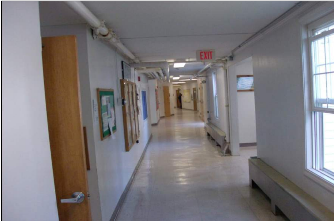
Note exposed sprinkler and heating pipes below ceiling.
