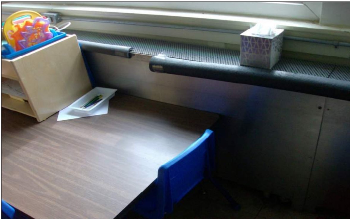
Fin tube radiators with vented covers.
