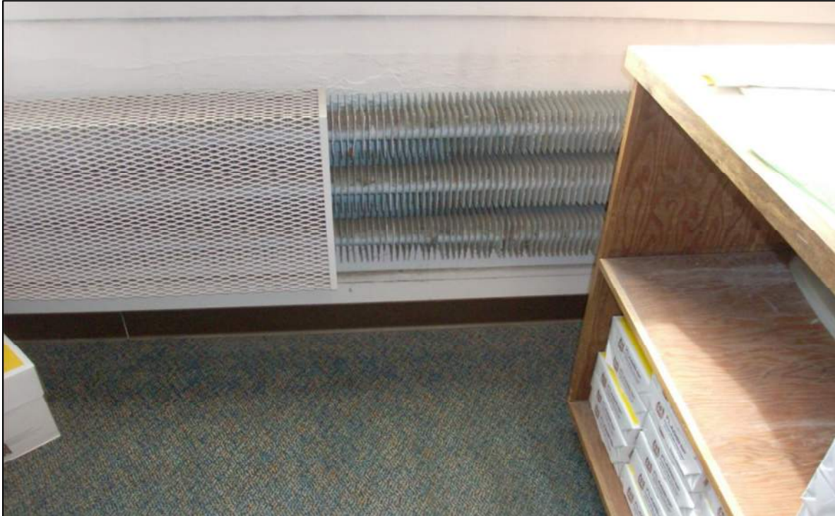
Typical fin tube radiators in older sections of school.
