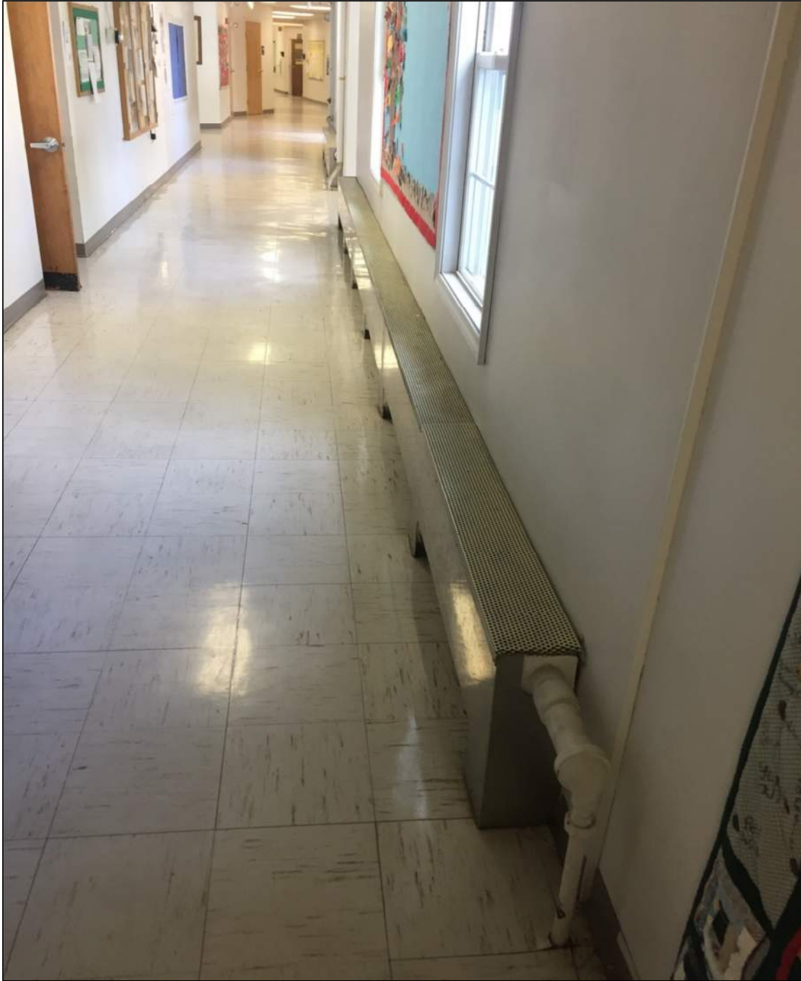
Fin tube radiators in corridor.
