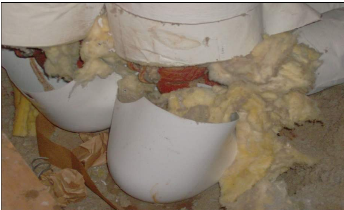
Original pipe insulation removed, but not properly replaced.
